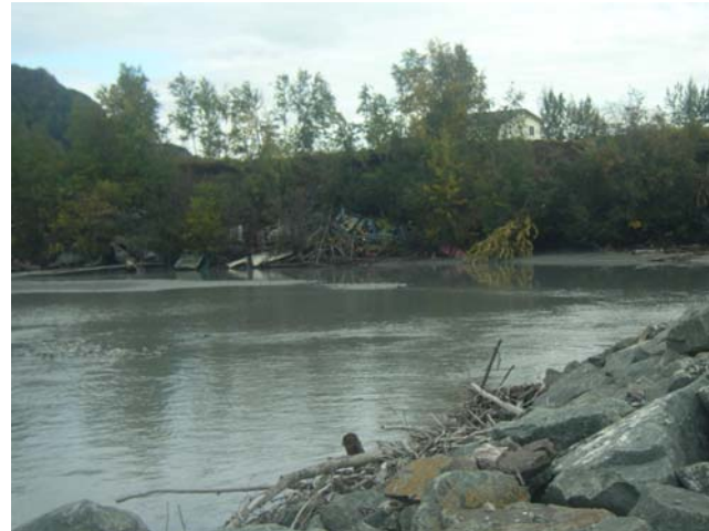
Photo 2: View from river end of Dike #5 Circle View Subdivision looking back at junk cars placed illegally to slow erosion, Sept. 2007.
