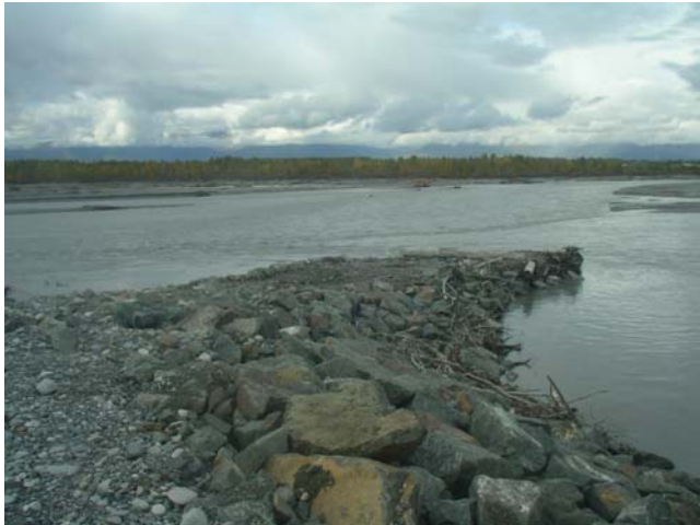
Photo 1: Finger dike #5 added in 2006 to protect lower end of Circle View Subdivision, Sept. 2007.
